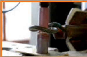
BRAZING COMPLETED WITHOUT OVER-SPILLAGE
